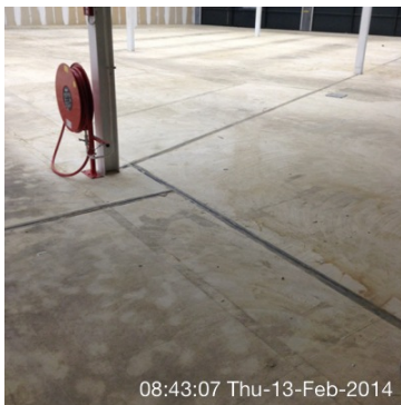
Expansion joint meeting centre of floor
