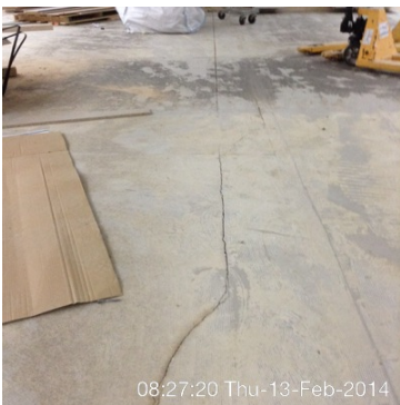
Movement joint screened over
